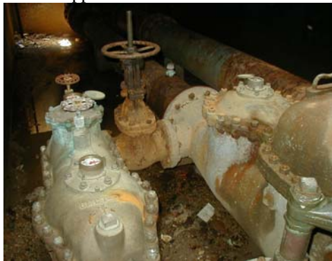
Meter Support Deficiencies
